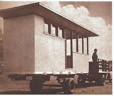
HOUSES—in mass production—from an assembly line! That's the feat just accomplished by the much-accomplished Tennessee Valley Authority. And now, from the TVA house-production factory, the factory-built, portable cottages are beginning to roll.
