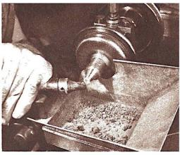
Above: After being cleaved, or sawed, the diamond is brought to the cutter, who rounds it, or puts a "girdle" on it. He gives it the approximate shape it will finally have. By a slight tap on the wheel he can cause the diamond to revolve irregularly, thus resulting in the desired shape. Another diamond is imbedded in the handle of the tool he uses. Right: Another view of the cutter at work. Only after years of practice is a man qualified to handle the precious stones.
