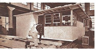
Here's the house assembly line. The cottage shown is almost completed, and the workman in the foreground is working on the floor platform of another.
