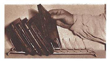
Left: A dish rack makes a handy film or plate holder file. Slots can be numbered and a record kept of the condition of film (whether exposed or not). loaded in each holder.—L. B. Robbins.
